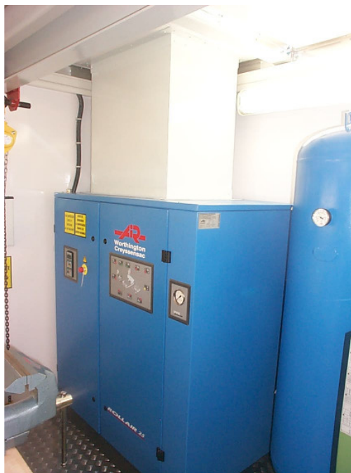
Screw air compressor
